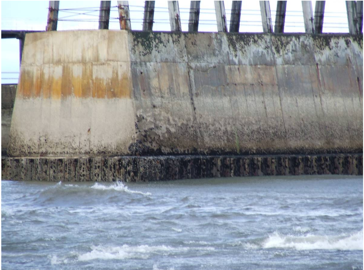
Figure 16 Landward End of East Pier Extension
