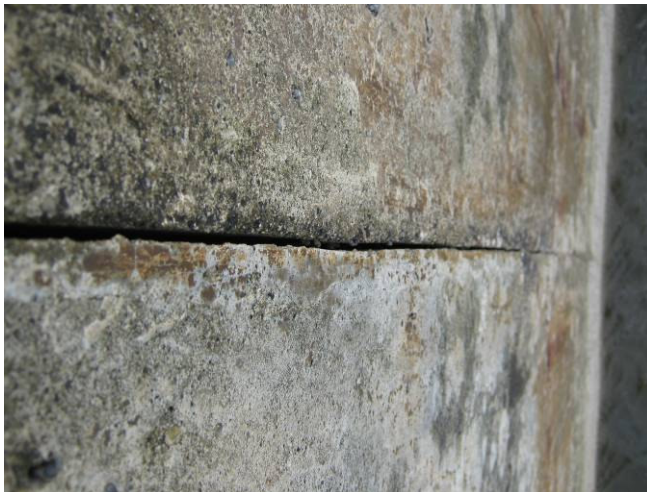
Figure 9 Vertical view down east face
